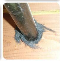
top of the basement wall for any light coming in. Plug any holes or cracks wider than  $\frac{1}{4}$ " with steel wool or steel wool and caulk to exclude mice. Or, you can install sheet metal flashing or hardware cloth over the crack or hole.
